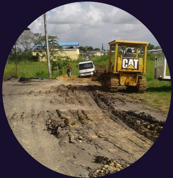
Breaking Ground in Trinidad
